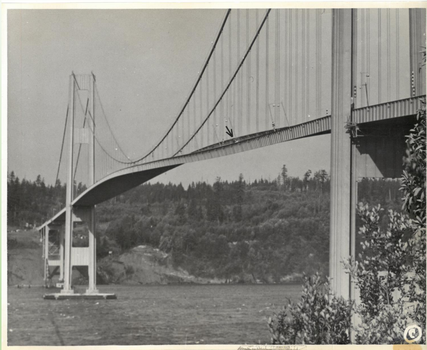
November 7, 1940, around 10am. Bridge undulating, the beginning of the collapse. An arrow drawn in the middle of the photograph points to the only car stuck on the bridge. Photograph taken from the embankment looking toward Gig Harbor. Photographer: James Bashford
