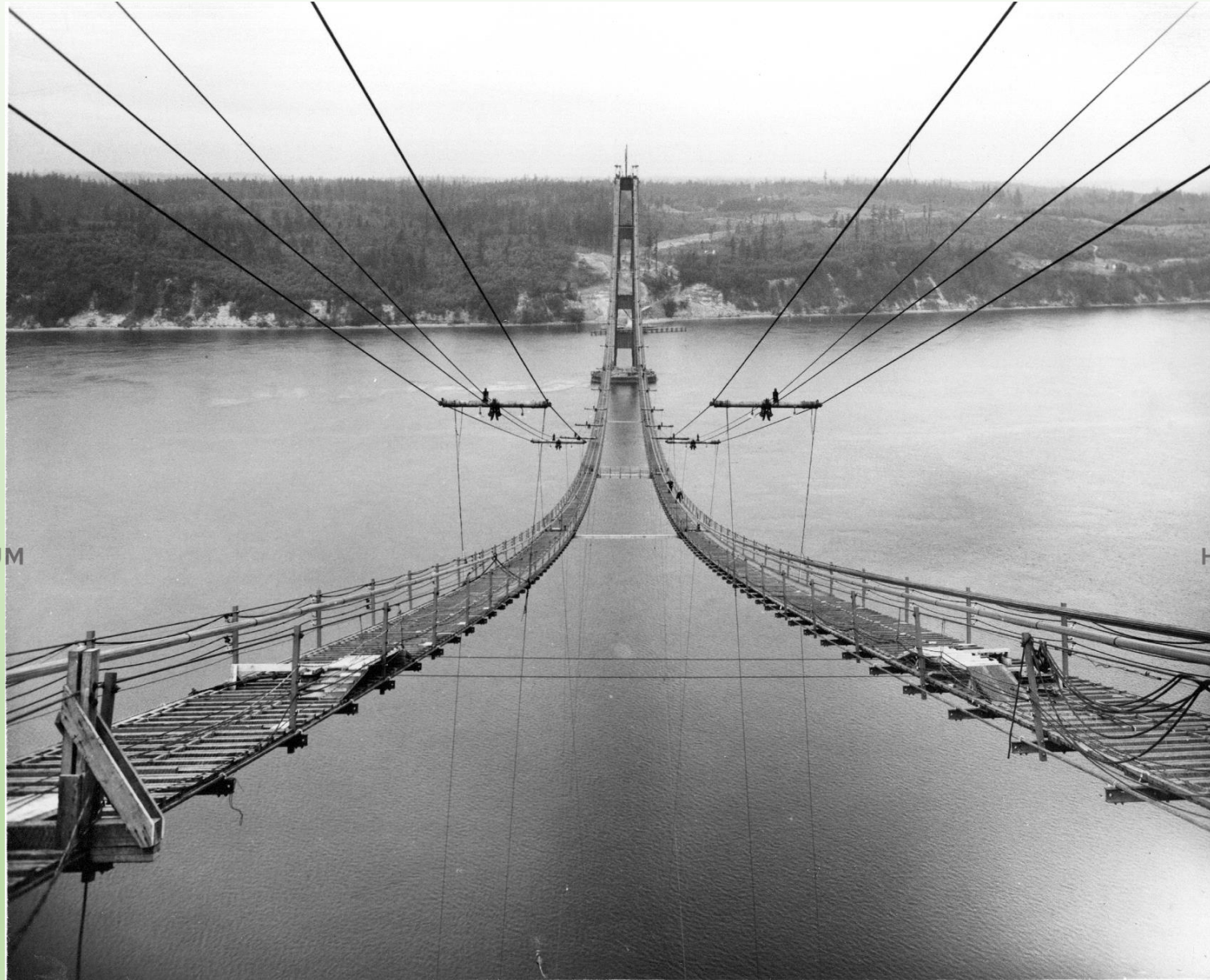
Catwalks were strung from the towers where the final suspension cables would hang. The cables that held the roadbed were hung from these main lines. 1938 – 1939. Photographer: James Bashford
