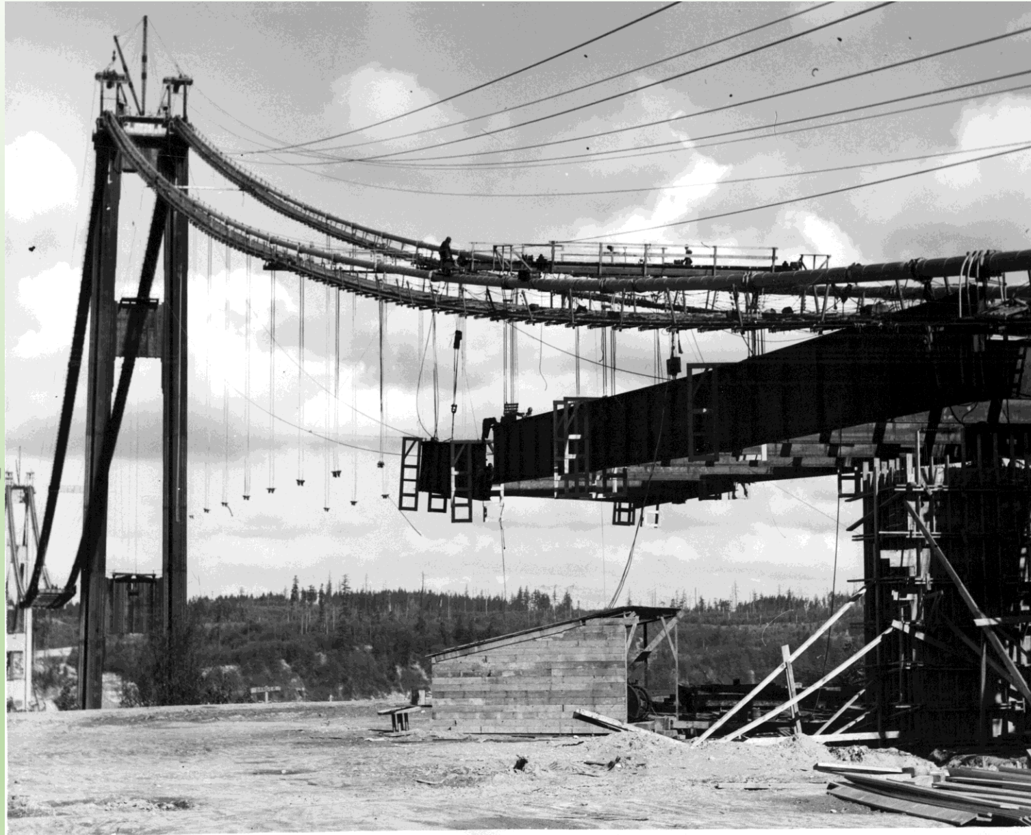
First Narrows Bridge under construction looking at the tower, part of the deck/roadbed, and part of catwalk. 1938 – 1939. Photographer: James Bashford
