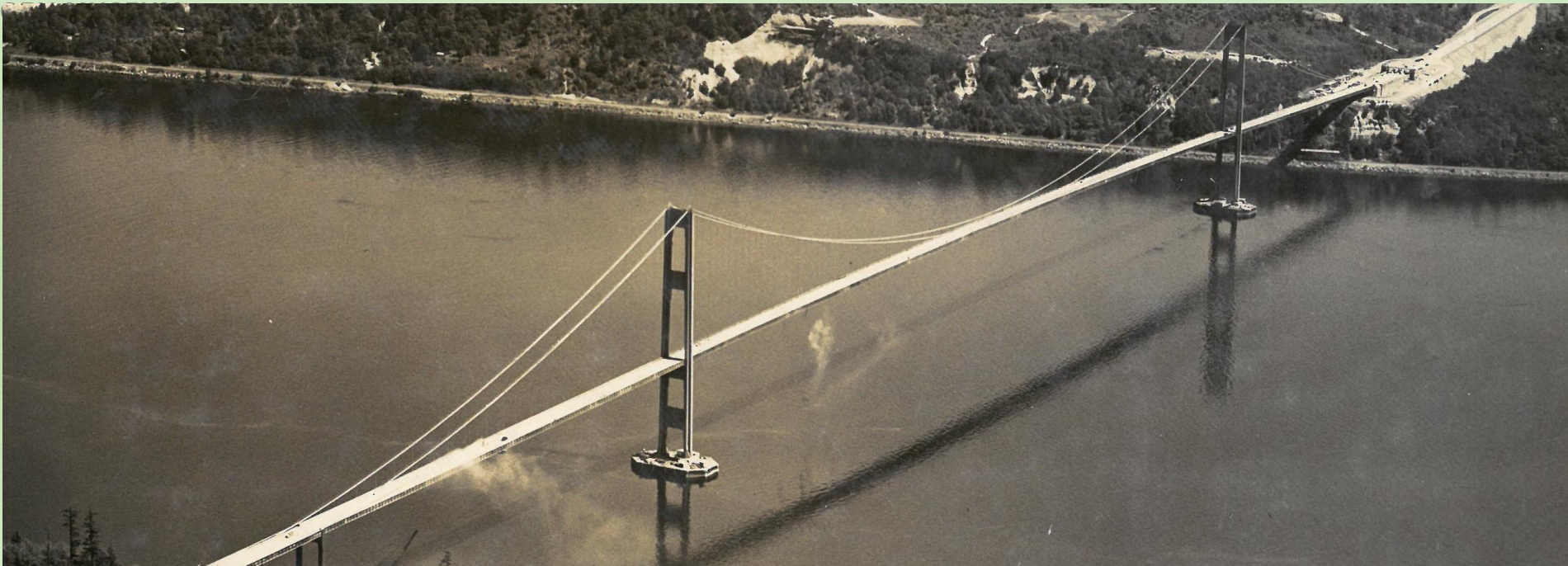
First Narrows Bridge, designed by Clark Eldridge and Leon Moisseiff, 1940. Photo by James Bashford
