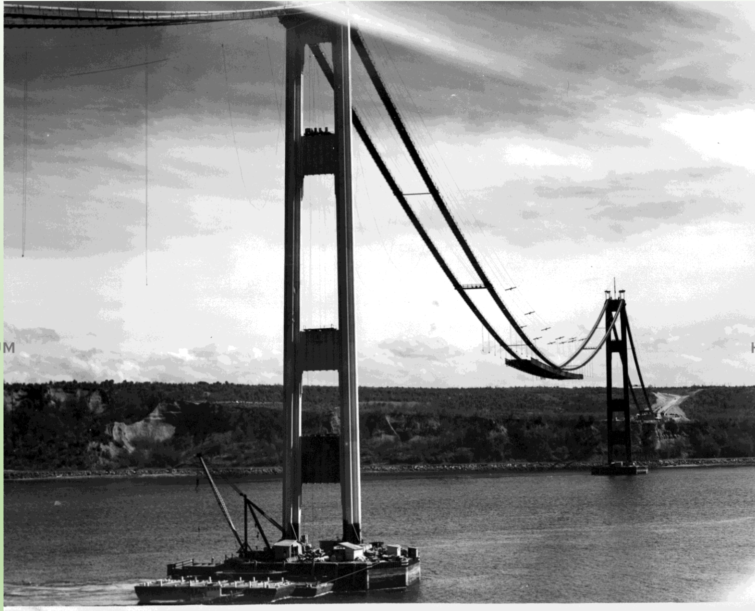
First Narrows bridge under construction. The first section of roadbed was attached to the lowest parts of the suspension cable. 1938 – 1939. Photographer: James Bashford
