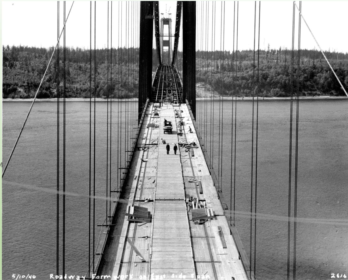
Construction of the first Narrows Bridge: Once the skeleton of the roadway was secured to the cables, concrete was poured to make a smooth, drivable surface. 1938 – 1939.
