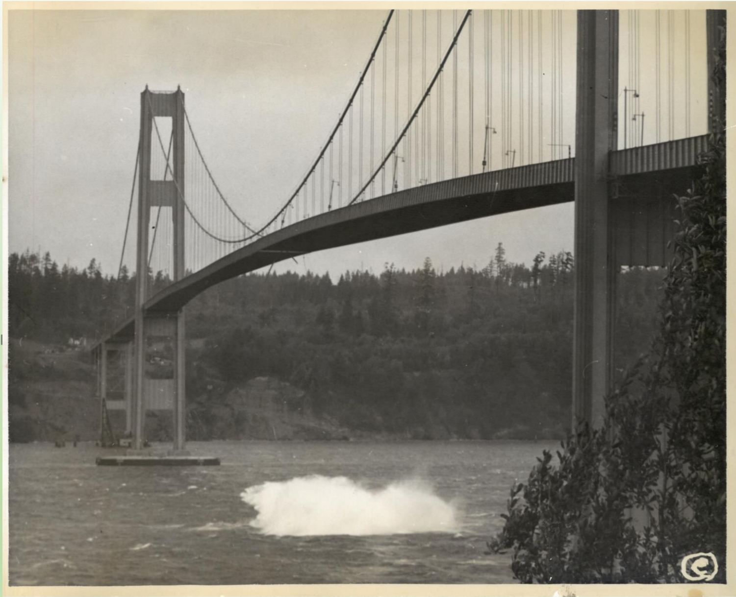
November 7, 1940, about 10:30 am. Bridge beginning to crack – a chunk of roadway splashes into the water. Photograph taken from the embankment looking toward Gig Harbor. Photographer: James Bashford
