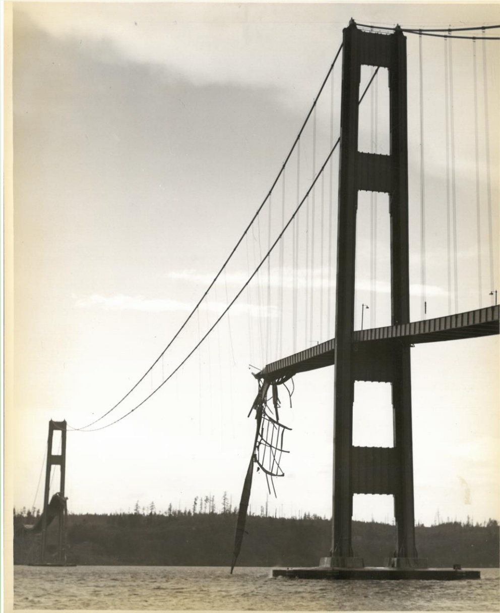
November 7, 1940, around 12 noon. Galloping Gertie with a shattered center span. A piece of gnarled deck dangles above the water. Photographer: James Bashford
