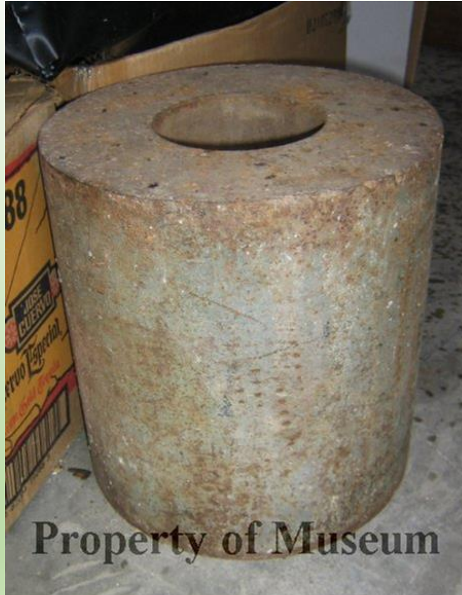
Cable spool from the first Narrows Bridge. Found by a scuba diver in the 1950s. Cable went through the hole in the middle of the spool. Height: 10.5 in, diameter: 10 in.
