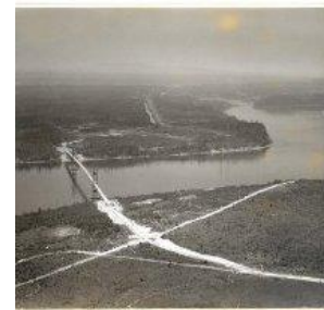
Object Name: Print, Photographic Date: 1940 Description: Aerial view of the Narrows bridge looking from University Place toward Gig Harbor. Roadway in Gig Harbor in the foreground. Photographer: Bashford, James Copyright: Photograph by James Bashford Collection: James Bashford Collection
